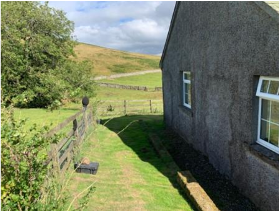
Figure C7 View of the monitoring location at 2 Byreclough Farm looking southeast
