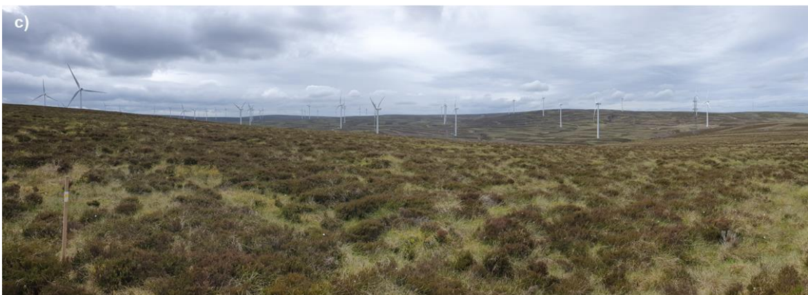
Plate 3.3 a) Typical heather dominated upland plateau in northern half of site, b) contrast between mature heather (foreground), muirburn (centre) and open grassy slopes in organic soils (left), c) Fallago Rig wind farm viewed from site
