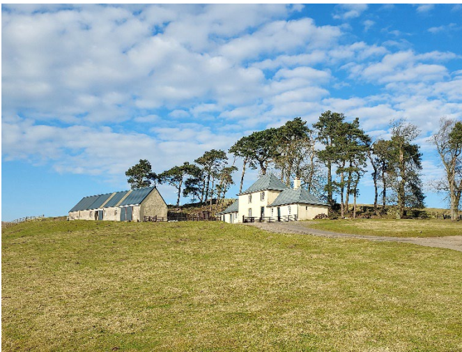
View looking north-west of Byrecleuch, Former Beater's Cottage (LB8348) and stables (SBC HER Ref: 15997)
